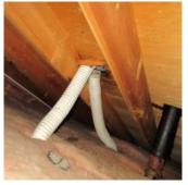
The ducts for exhaust fans in the bathrooms were vented to a box vent in the attic.
