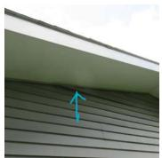
The exterior was vinyl siding. It was in good condition. There was one piece that the channel had separated. It should be locked together.
